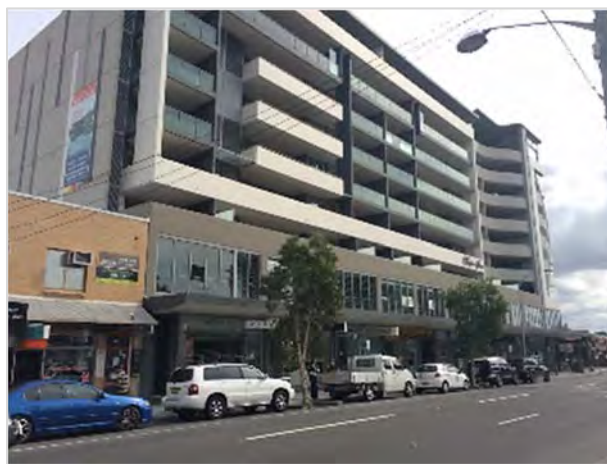
Figure 8: looking west on Bay Street
