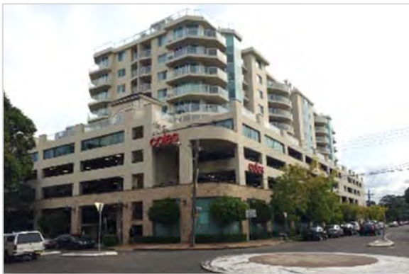
Figure 13: Development to the west, looking west on Princess Street.
