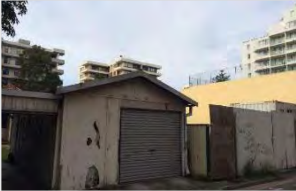
Figure 11: Looking north east on Saywell Lane at the rear of 16-20 Princess Street.
